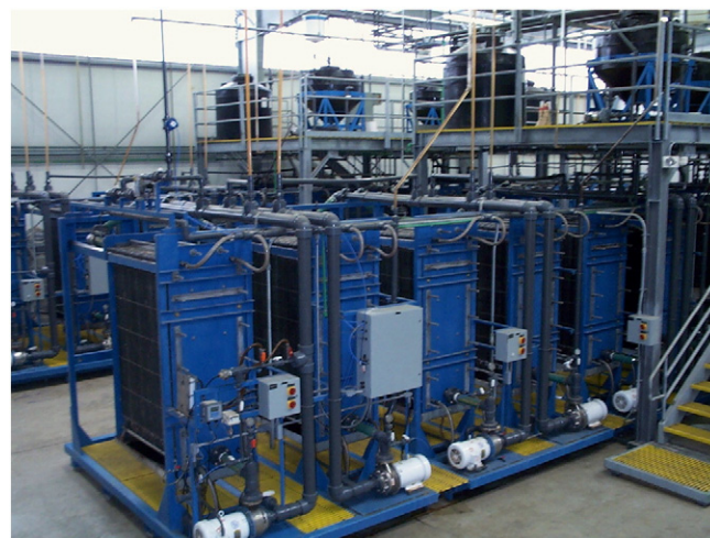
Fig. 7. Full-scale plate-and-frame FO treatment system operated at Coffin Butte Landfill by HTI (previously Osmotek) for treatment of landfill leachate.
